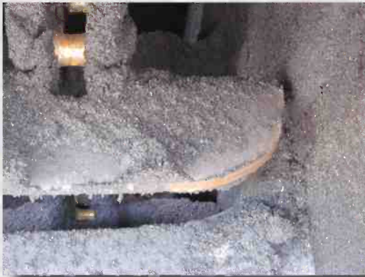
Heavy corner wear on slats and asphalt buildup causes high wear on chains and sprockets
